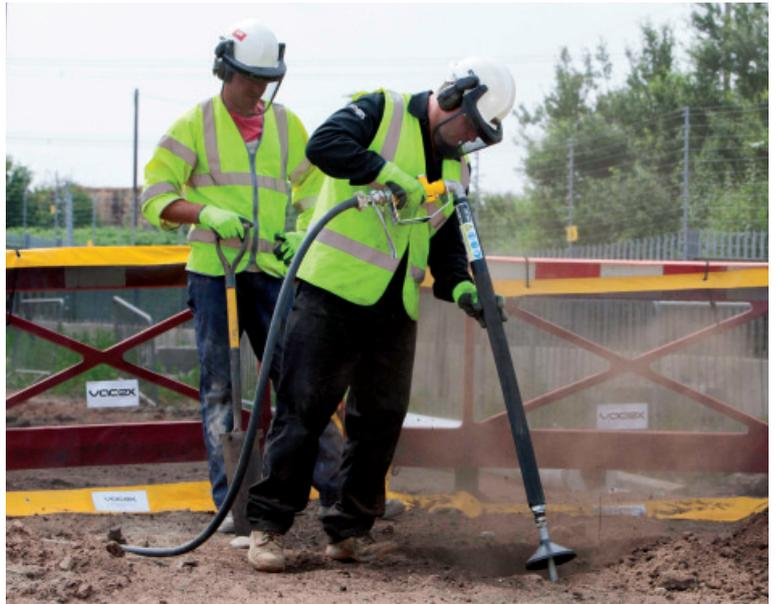
The **Air-Ex** system is the safest way to remove material from unknown utilities, obstructions and tree roots, being non-aggressive and non-invasive.
